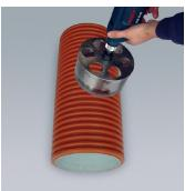
2- Reverse hole-saw softly to avoid damage and use a sandpaper to eliminate rough edges and particles. Wipe area clean removing all debris from inside the pipeline and around the joint face.
